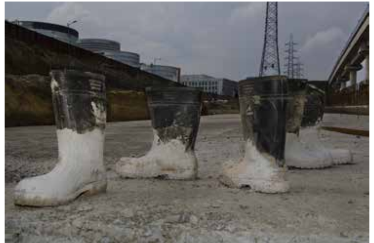
Workers' gumboots seen at an empty IL&FS construction site for the DLF underpass.
