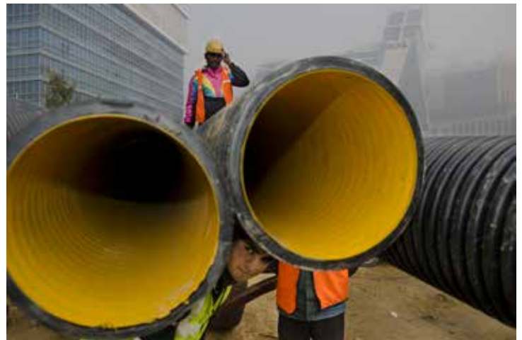
Workers at an IL&FS construction site near Cyber City.
