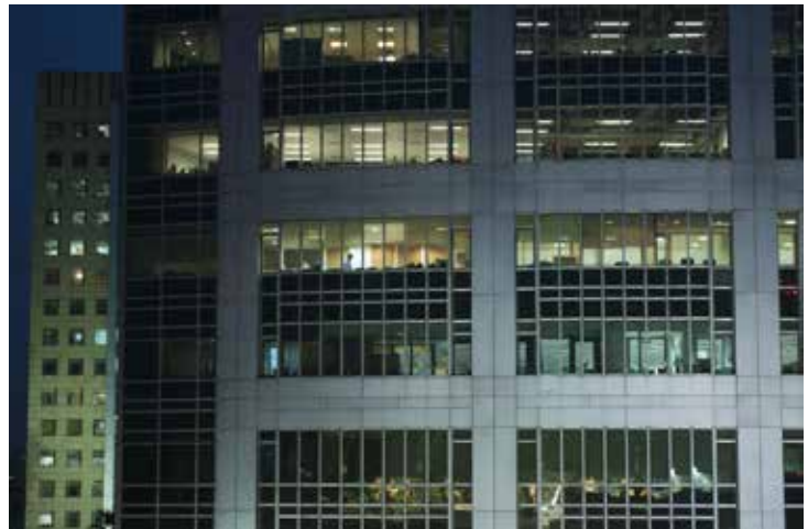
A view of a corporate office by night from a metro station.
